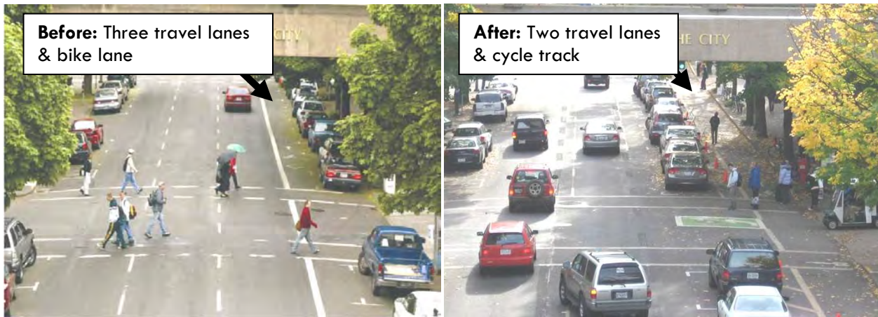
Figure 3. SW Broadway, Before and After Cycle Track Installation
