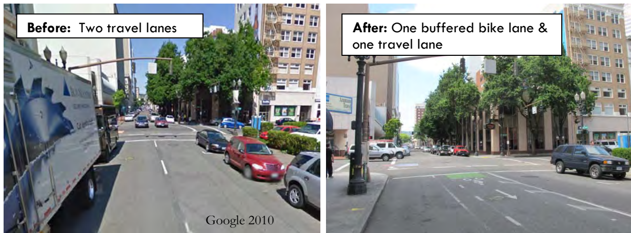
Figure 5. SW Stark at 4 th Avenue, Before and After Buffered Bike Lane Installation
