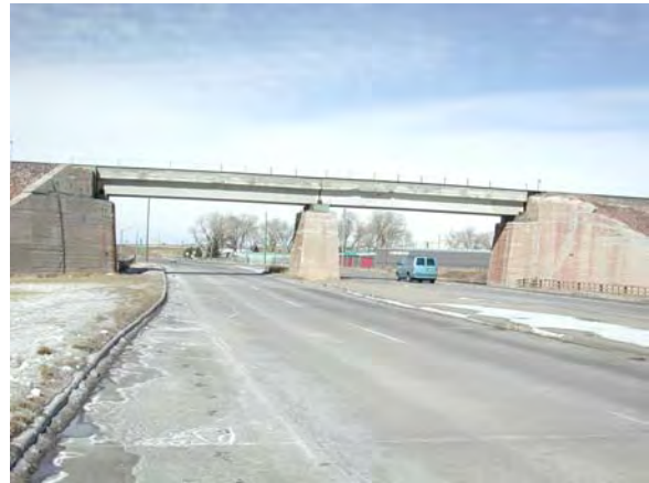
Railway crossing over Missile Drive
