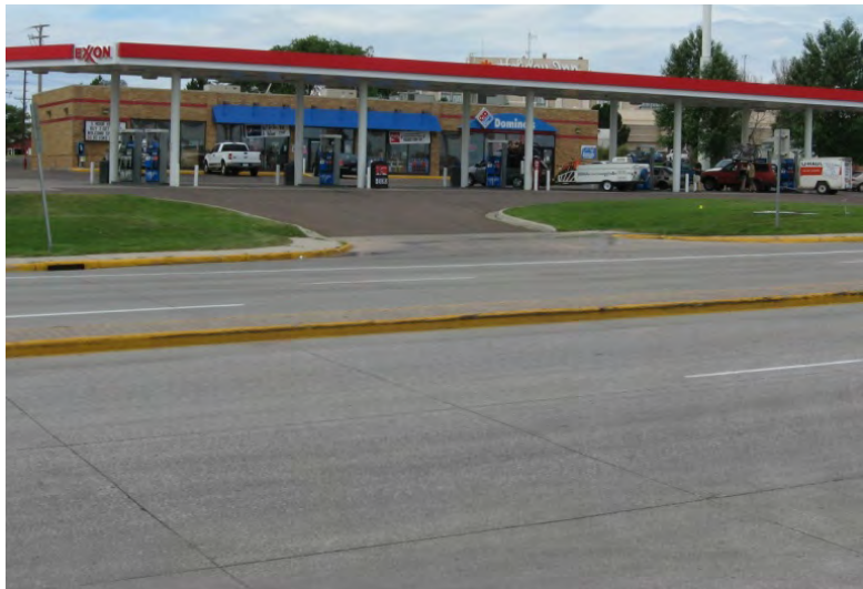
Existing raised median along SGH north of Fox Farm Road
