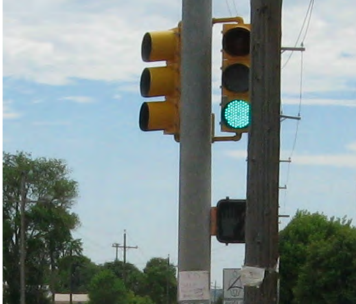
Photo 2 - Utility pole blocking view of “Walk” signal
