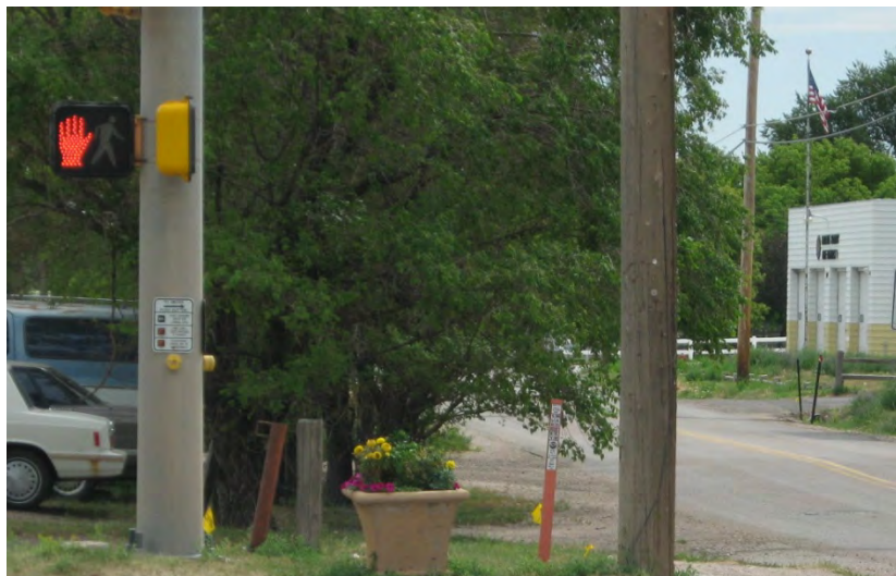
Photo 1 -Pedestrian push button out of reach from sidewalk, particularly for physically impaired users
