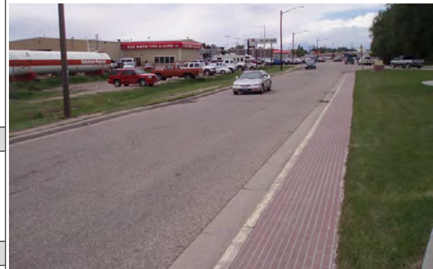
The eastbound “slip lane” on East Lincolnway facilitates high vehicle speeds and difficult pedestrian crossing conditions.
