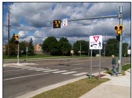
Figure 58. HAWK signals, such as this one located in West Bloomfield Twp, Michigan) can improve crossing conditions at locations where a full signal is not needed
