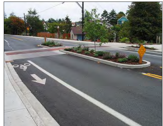
Figure 45. Example of a pedestrian refuge island
