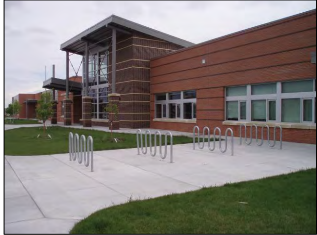
Figure 42. Sunrise Elementary offers 'wave rack' style bicycle parking and excellent ADA accommodation on school grounds
