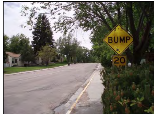
Figure 7. Overgrown vegetation impedes pedestrian travel on sidewalks
