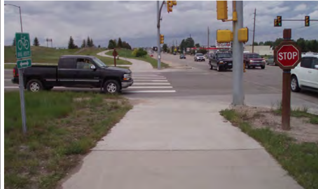
Installation of stop lines can provide visual guidance for motor vehicles on where to stop and help keep crosswalks clear for bicyclists and pedestrians.
