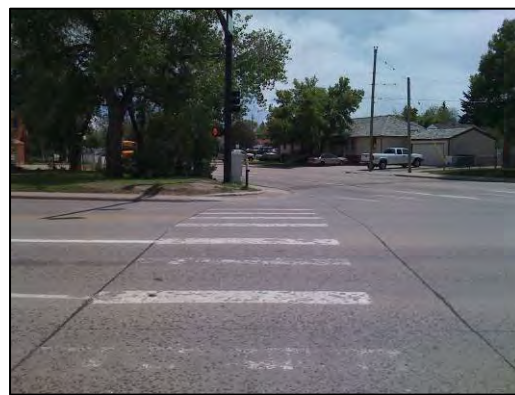
Figure 9. Faded crosswalks can be hazardous to pedestrians
