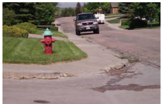
Figure 11. Older curb ramps typically have a greater cross and running slope than the maximum allowed by current ADA standards.
