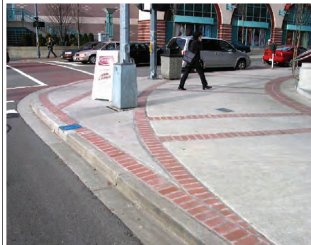
Figure 21. This corner was reconstructed to reduce vehicle turning speeds and to provide additional pedestrian space.
