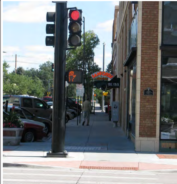
Figure 10. Example of a curb ramp with truncated domes.
