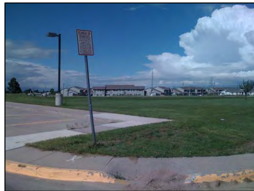
Figure 12. Curb ramps with steep grades, and/or poor maintenance can render a sidewalk inaccessible to a pedestrian in a wheelchair
