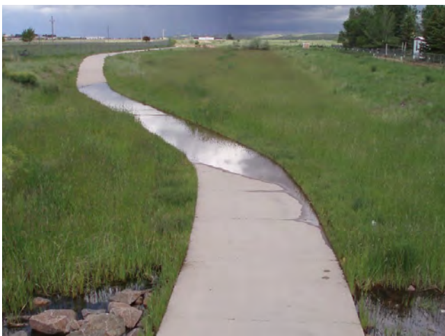
Figure 25. Heavy rainfalls can flood existing Greenways. Water or ice on the trail can further discourage pedestrian use.
