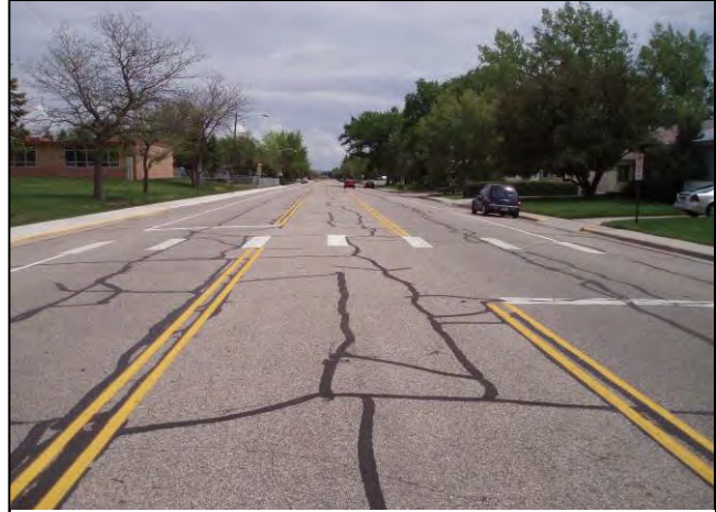
Figure 34. The mid-block crossing of Henderson Avenue lacks curb ramps, creating accessibility challenges for pedestrians with physical disabilities
