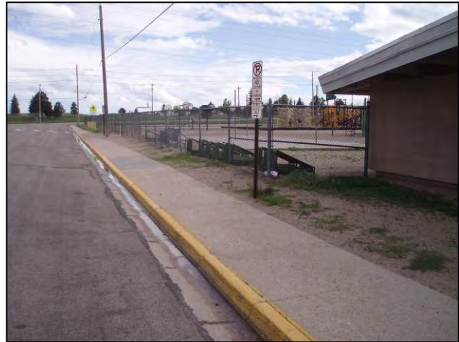
Figure 32: The school bus and student load zones at Goins Elementary lack Advance Warning signage
