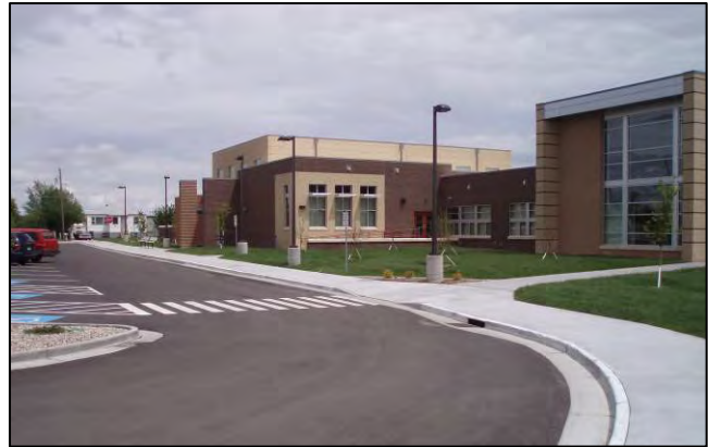
Figure 21. Baggs Elementary School has a pedestrian friendly environment that includes wide sidewalks, crosswalks, and curb ramps.
