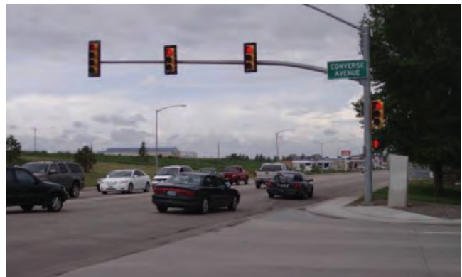
Figure 13. Intersections along Converse Avenue have pedestrian signal heads and ADA-compliant curb ramps.
