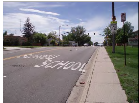
Figure 52. School pavement markings
