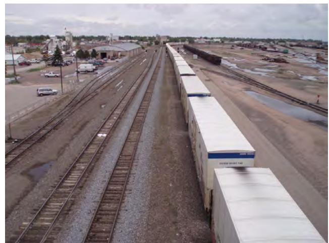
Figure 23. The UPRR rail yard creates a significant barrier between downtown and southern Cheyenne.
