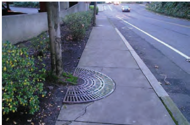
Figure 16. Tree well grates should be flush with the sidewalk surface.
