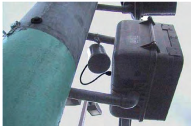
Figure 24. Speaker on pedestrian traffic signal
