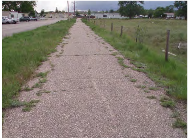
Figure 26. Aging and deteriorated walkways create uneven travel surfaces.
