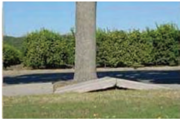
Figure 15. Subsurface tree roots can lift concrete sidewalk slabs, causing the surface to become uneven.
