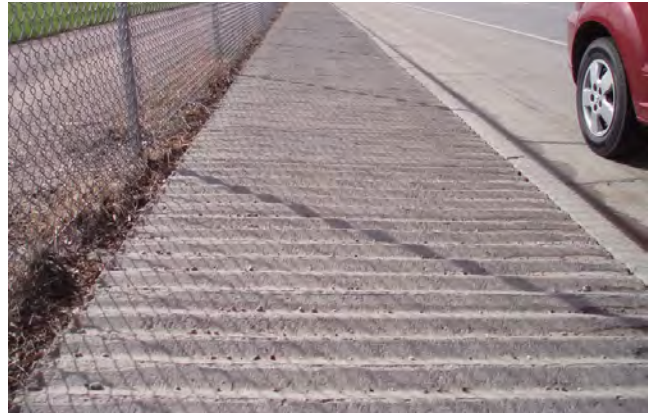
Figure 7. Ridged sidewalks along Yellowstone Road create challenging and uncomfortable travel conditions for pedestrians.
