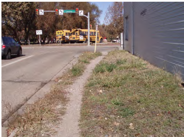
Figure 27. Demand paths alongside roadways indicate the need for formalized pedestrian facilities.
