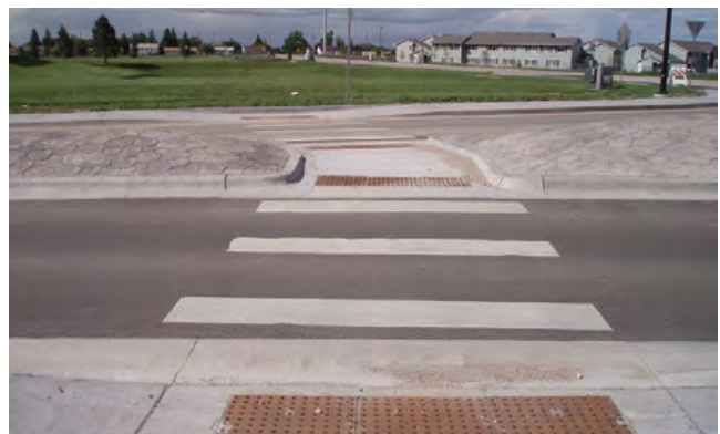
Figure 15. The modern roundabout at Snyder Avenue and Allison Road provides crosswalks and signage on all approaches.
