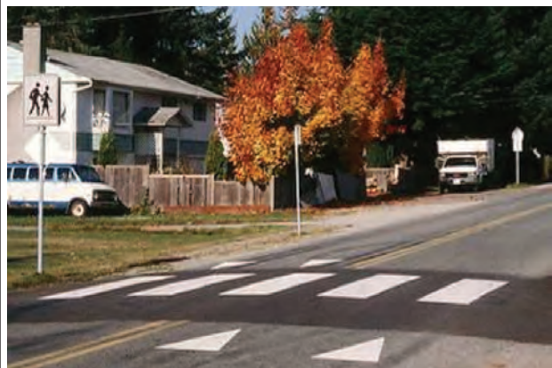
Figure 33. Raised crosswalks increase pedestrian visibility. Source: www.walkinginfo.org
