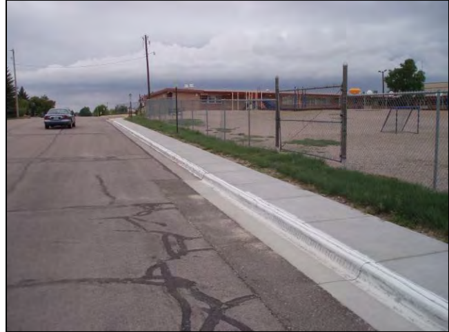
Figure 23. Narrow sidewalks near Buffalo Ridge Elementary
