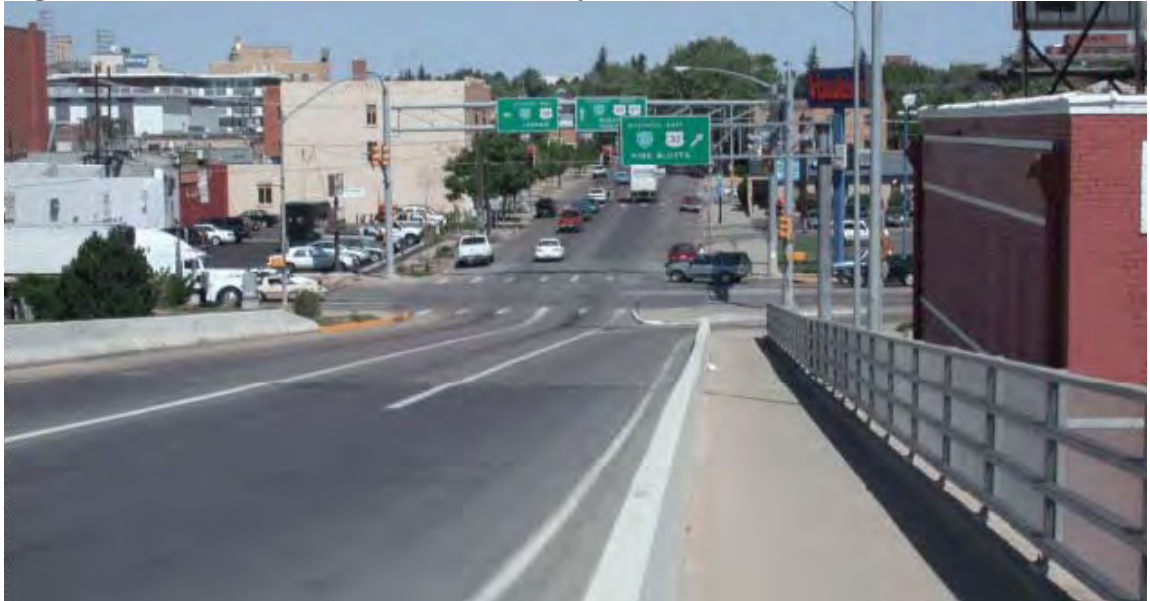
Figure 2. Northbound I-180 at Lincolnway
