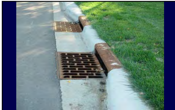
Better solution: indent grates into the planter strip
