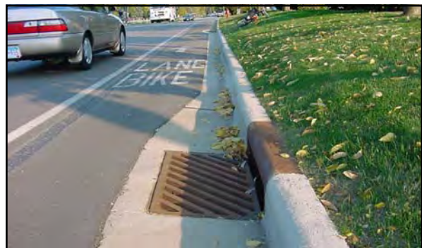
Drainage grates are often wider than the normal gutter – one solution is to expand the gutter width
