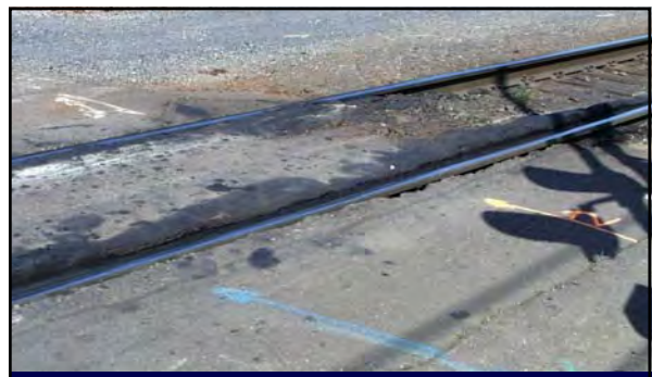
Wide flange opening can trap wheels
