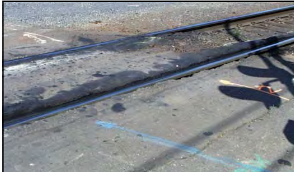
Crossing materials: Asphalt – OK at first ,but must be maintained
