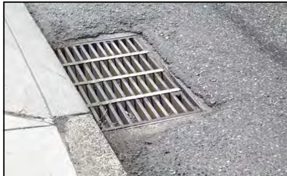
Retrofit – weld straps transverse to bicycle travel
