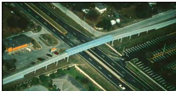
Overcrossing: long ramps can be placed in line with the trail
