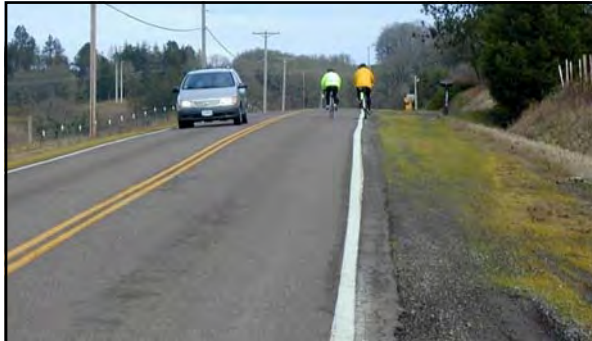
Shared roadway common and appropriate on rural back roads
