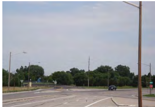
MISSILE DRIVE APPROACHING 19TH STREET INTERSECTION
