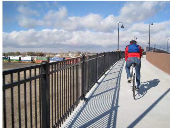
Figure 17. Barriers, such as the Union Pacific Railroad tracks, can be overcome by constructing facilities like the Greenway extension on the Norris Viaduct.
