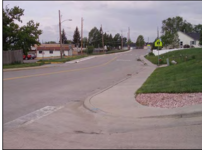
Figure 26. Pavement Markings and Advance School Warning Signs on Montclair Drive
