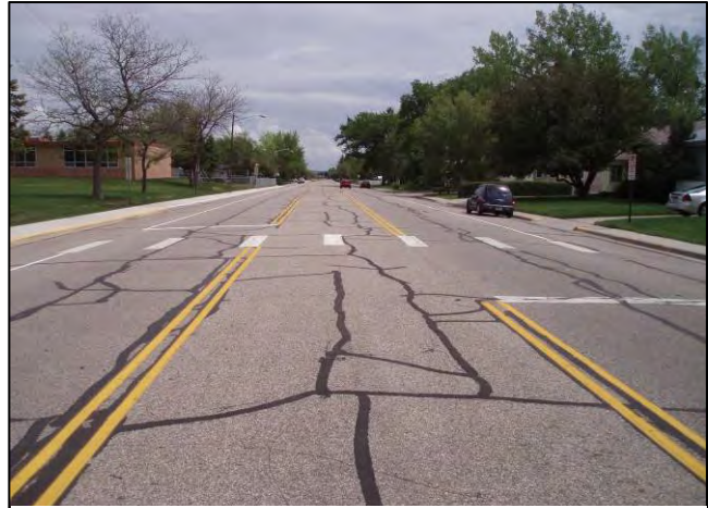
Figure 34. The mid-block crossing of Henderson Avenue lacks curb ramps, creating accessibility challenges for pedestrians with physical disabilities
