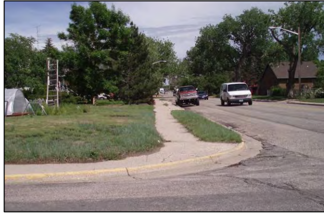
Figure 28. Narrow sidewalks without curb ramps characterize the area around Deming Elementary
