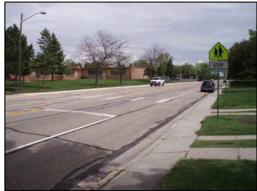
Figure 59. Stop lines, or yield lines provide guidance for motorists about the desired stop location when a crosswalk is occupied.
