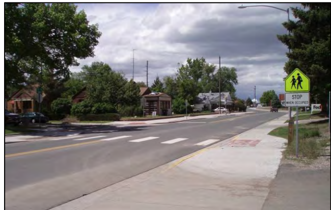
Figure 27. A school crossing near Miller Elementary School has a stop line for southbound vehicles, enhancing pedestrian safety and comfort
