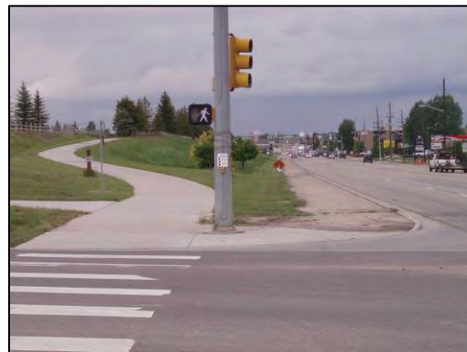
Figure 10. Well-marked crosswalk with pedestrian push-button
