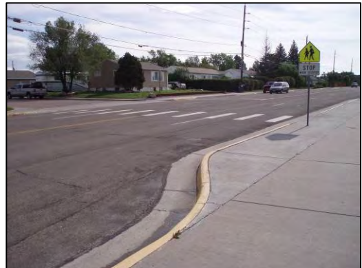
Figure 55. Curb extensions reduce the required crossing distance at some designated school crossings
