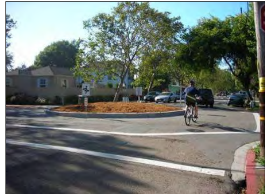
Figure 49. Traffic circles are one method of creating a pinch point
