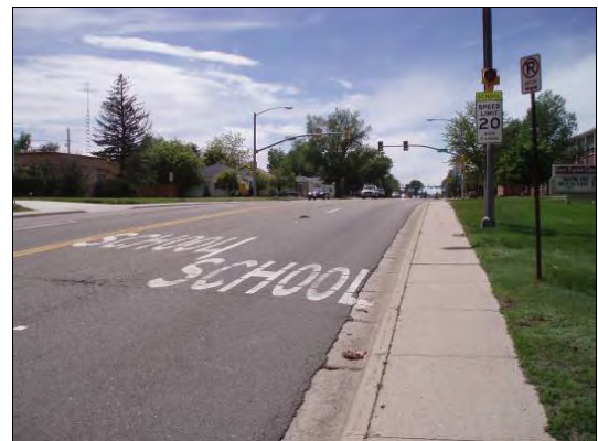
Figure 52. School pavement markings
