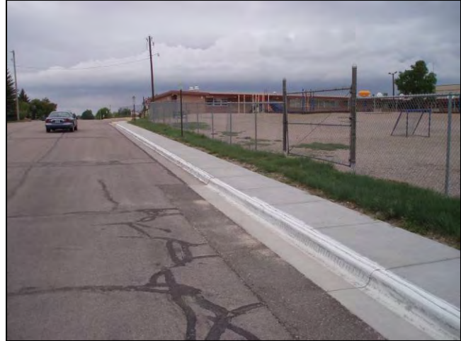
Figure 23. Narrow sidewalks near Buffalo Ridge Elementary
