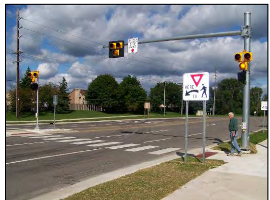
Figure 58. HAWK signals, such as this one located in West Bloomfield Twp, Michigan) can improve crossing conditions at locations where a full signal is not needed
