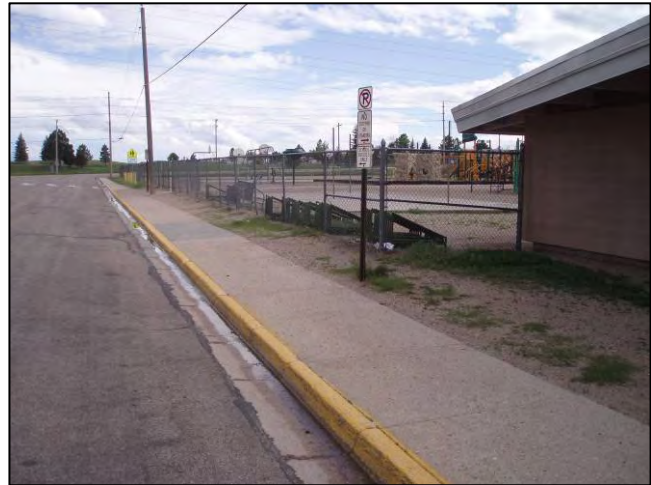
Figure 32: The school bus and student load zones at Goins Elementary lack Advance Warning signage
