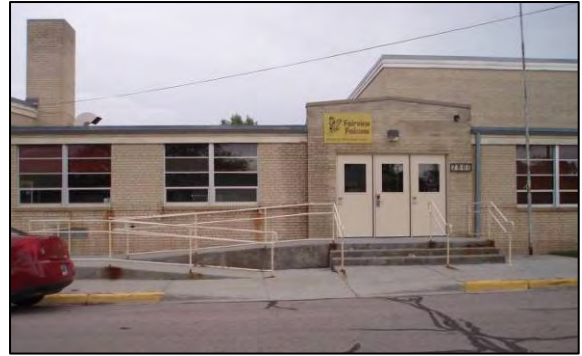
Figure 30. Access to the school grounds at Fairview Elementary is generally adequate
