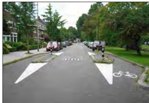
Figure 48. Paired chicanes create a pinch point that narrows roadway width and slows traffic
