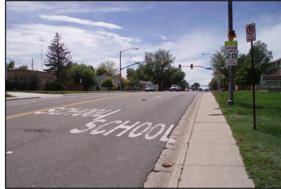
Figure 24. Warning signs, pavement markings and pedestrian actuated signals aid pedestrian crossings of Pershing Boulevard
