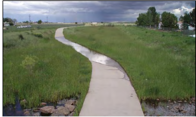
Figure 17. Students utilizing the greenway system may encounter pathway flooding during the rainy season
