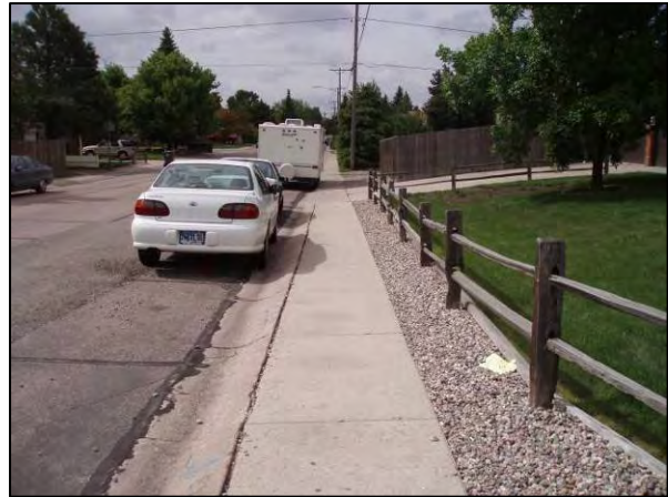
Figure 35. Narrow sidewalks near Hobbs Elementary
