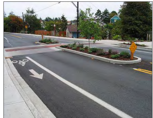
Figure 45. Example of a pedestrian refuge island
