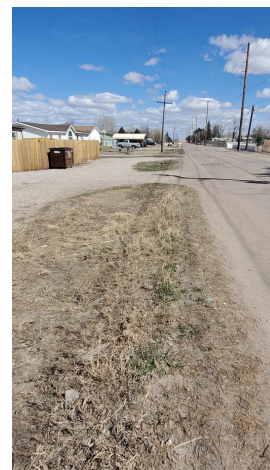
OPEN DITCH ALONG NORTH SIDE OF EAST ALLISON
