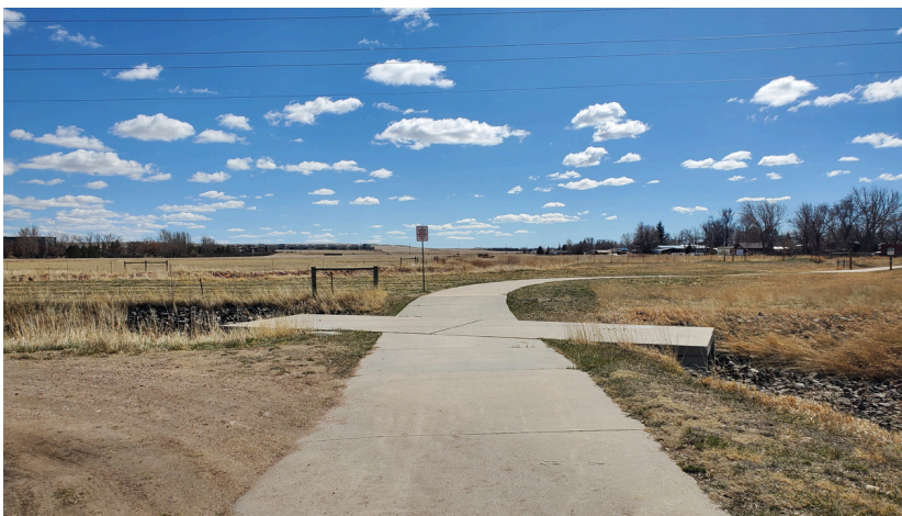
CULVERT TO ALLISON DRAW
