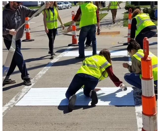
Figure 42: Pop-up Crosswalk for Safety and Neighborhood Connection (Credit: Active Wisconsin)
