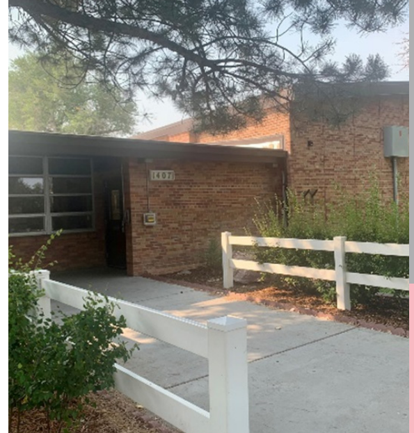
Figure 124: Pioneer Park Street View
