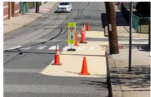
Figure 43: Painted curb bumpouts (Credit: City of Somerville)
