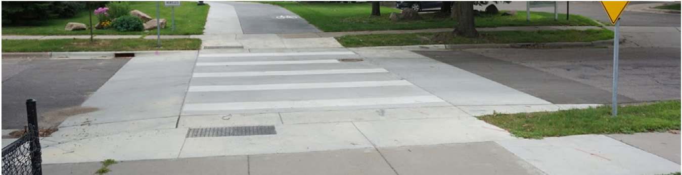
Figure 51: Raised pedestrian and bicycle crossing (Credit: City of Minneapolis)
