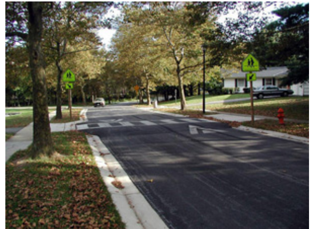
Figure 52: Raised crosswalk (Credit: Pedestrian and Bicycle Information Center)
