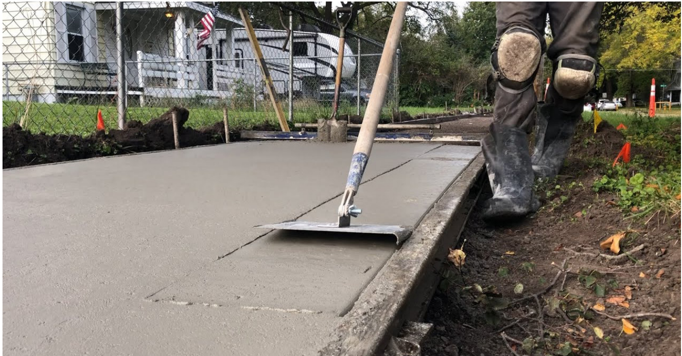
Figure 57: Sidewalk construction (Credit: City of Des Moines)
